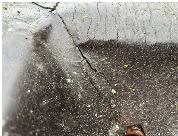
Foto 5.4: Scheur in de dakbedekking in de hoek
